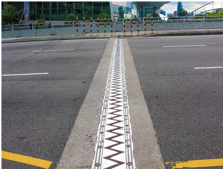
**Figure 1. Expansion Joint on a Bridge in Order to Prevent Cracking**
