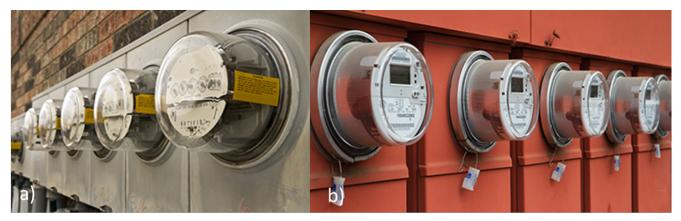
Figure 1. Electromechanical Meters (a); and E-meters (b)
