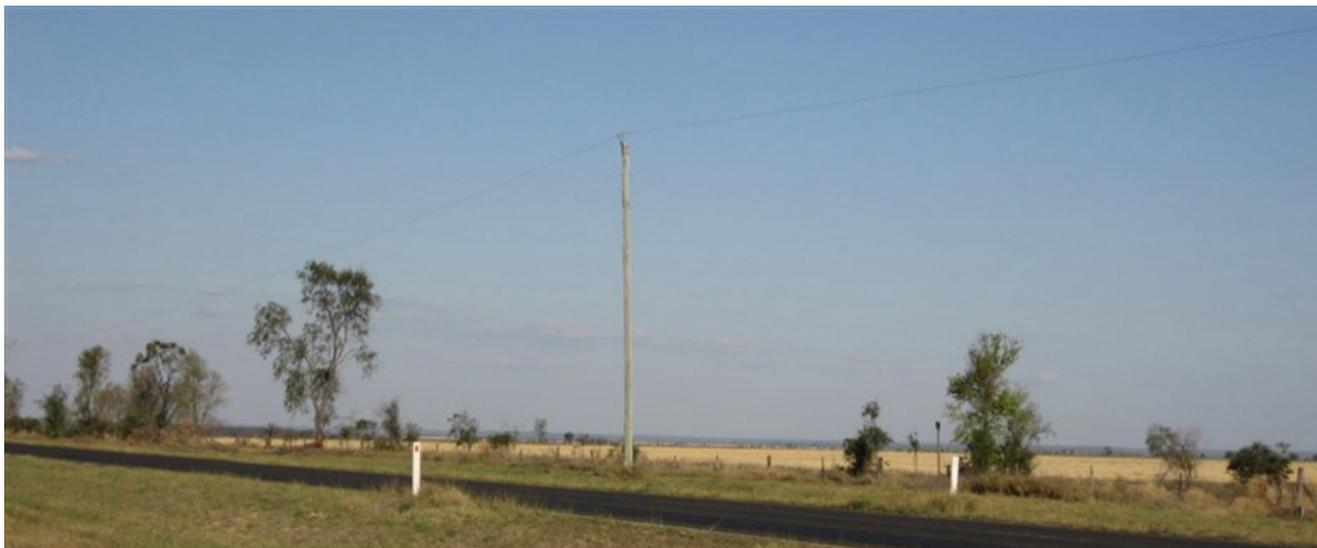
**Figure 1. A SWER Transmission Line Using a Single Wire to Connect a Rural Community to the Network**
